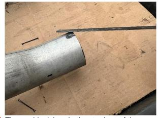
29. Thoroughly deburr both cut edges of the FACTORY REAR MUFFLER exhaust section.
